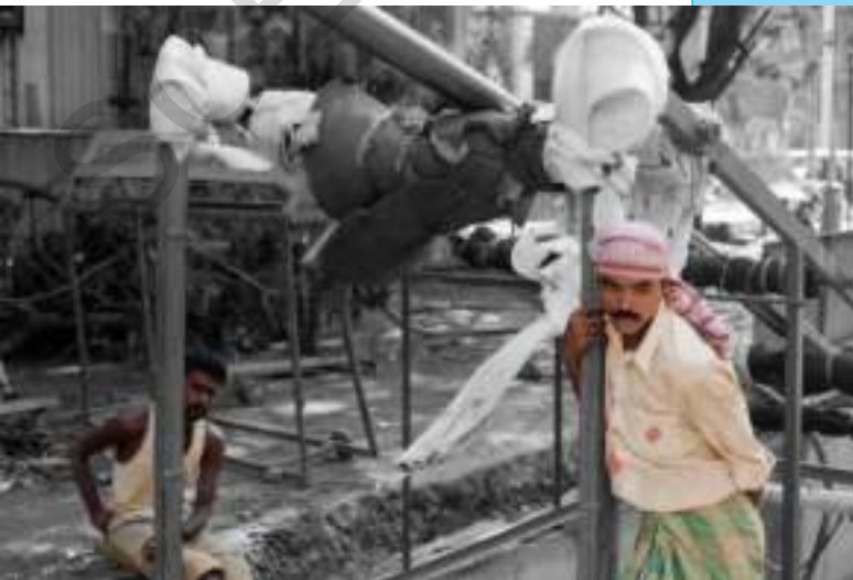
Fig 19.5 Road Laying Work
