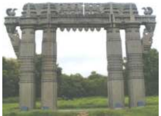
Fig 12.1 Kirti Torana entrance of Svayambhu Siva Temple - built by Kakatiya kings in Warangal.
