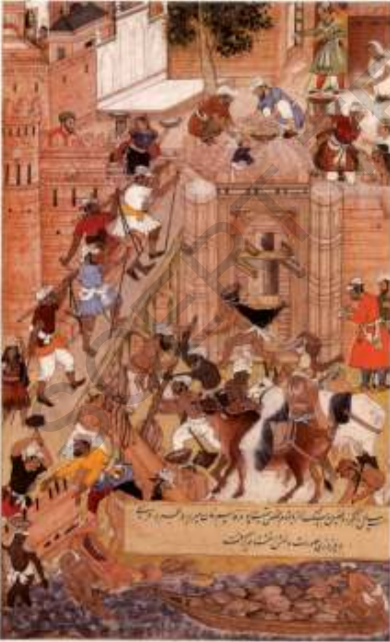
Fig: 22.6 A painting from the Akbar Nama (dated 1590-1595), showing the construction of water gate at Agra Fort.
