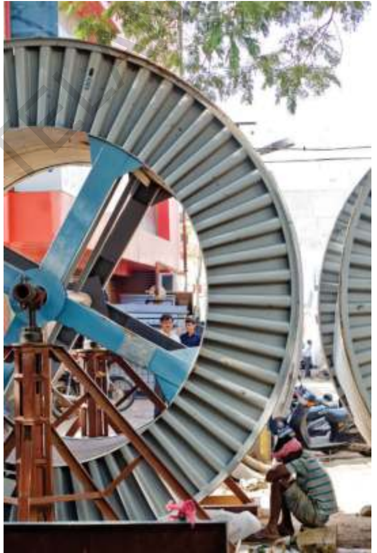
Fig 19.4 Workers laying cables
