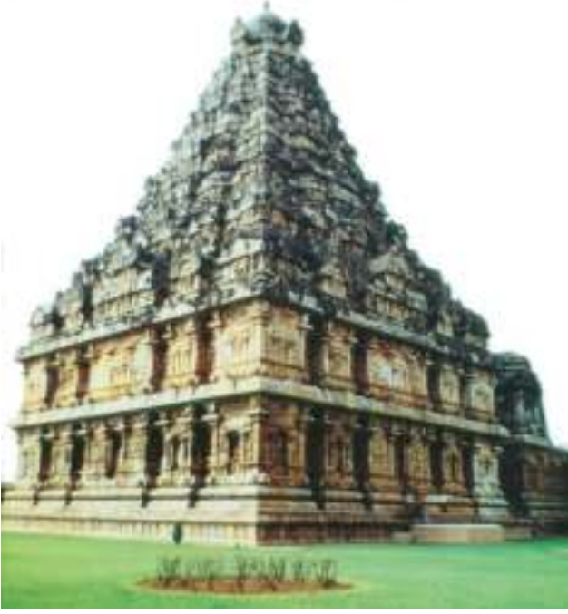
Fig 11.3 The temple at Gangaikonda-Cholapuram. Notice the way in which the roof tapers. Also, look at the elaborate stone sculptures used to decorate the outer walls
